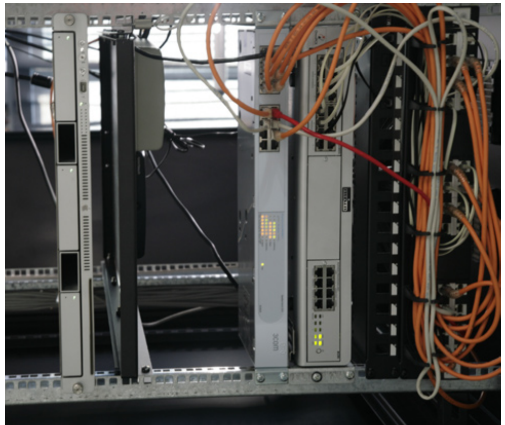
Here is a detail of the large Macintosh server module. CCG has heavy duty equipment in every respect.
