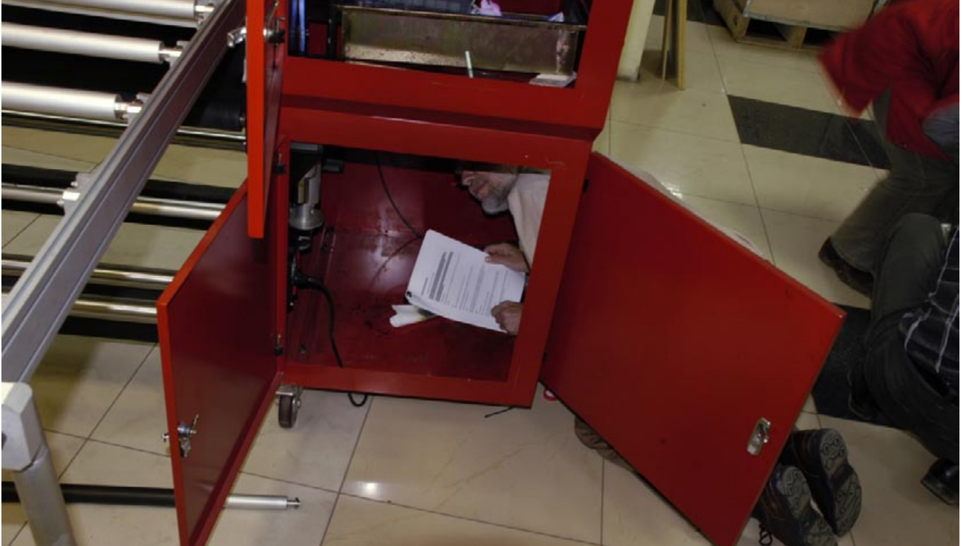
The photo above shows me inside inspecting the welds. You can't do this at a trade show.
