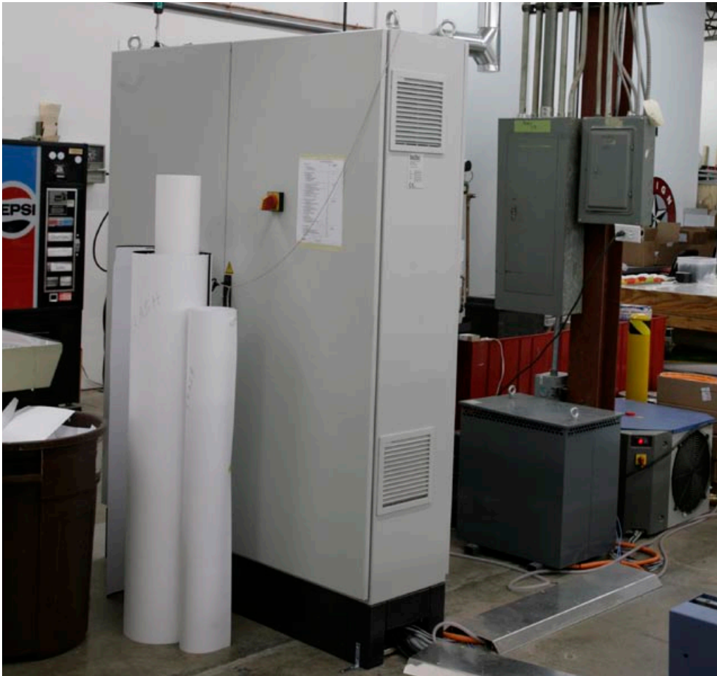
Sample of how much electricity an over-sized UV flatbed required: Luscher JetPrint electrical unit, at site-visit case study near the FLAAR office in St Louis, Missouri.
