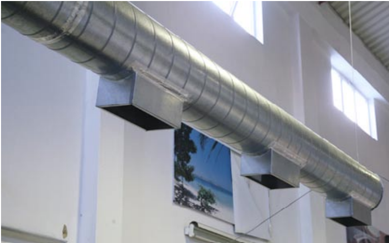
Exhaust system installed inside the facilities to avoid VOC and other hazardous elements from accumulating. Gandiinnovations site visit in Lisbon, Portugal.
