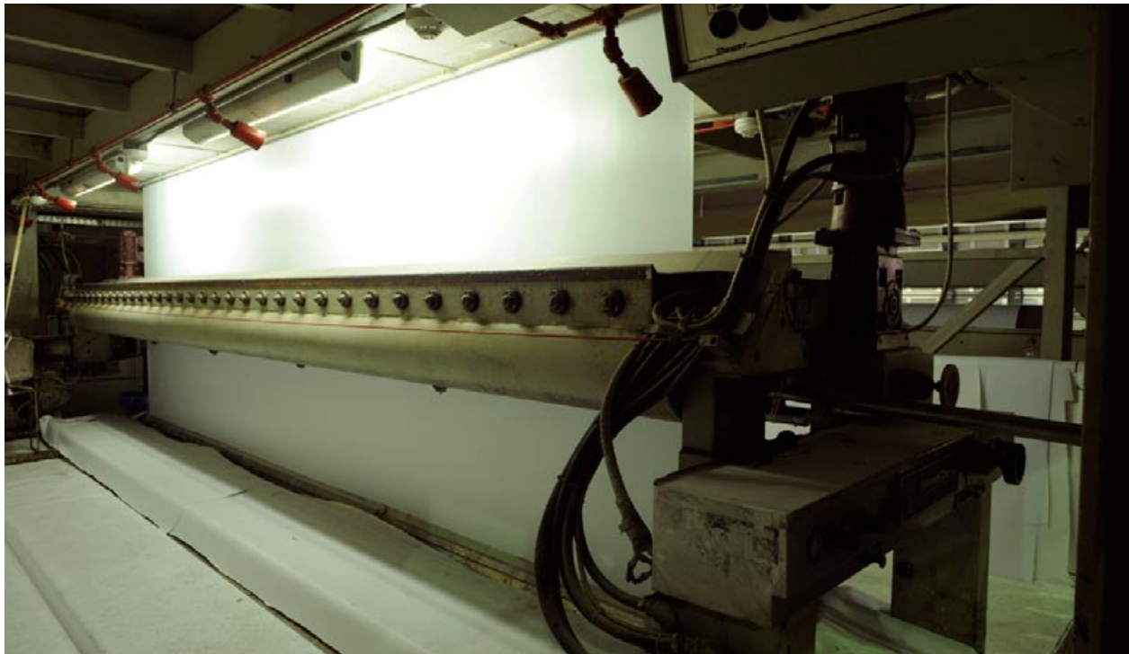
Here you see inside the 5-meter PVC coating mill.
