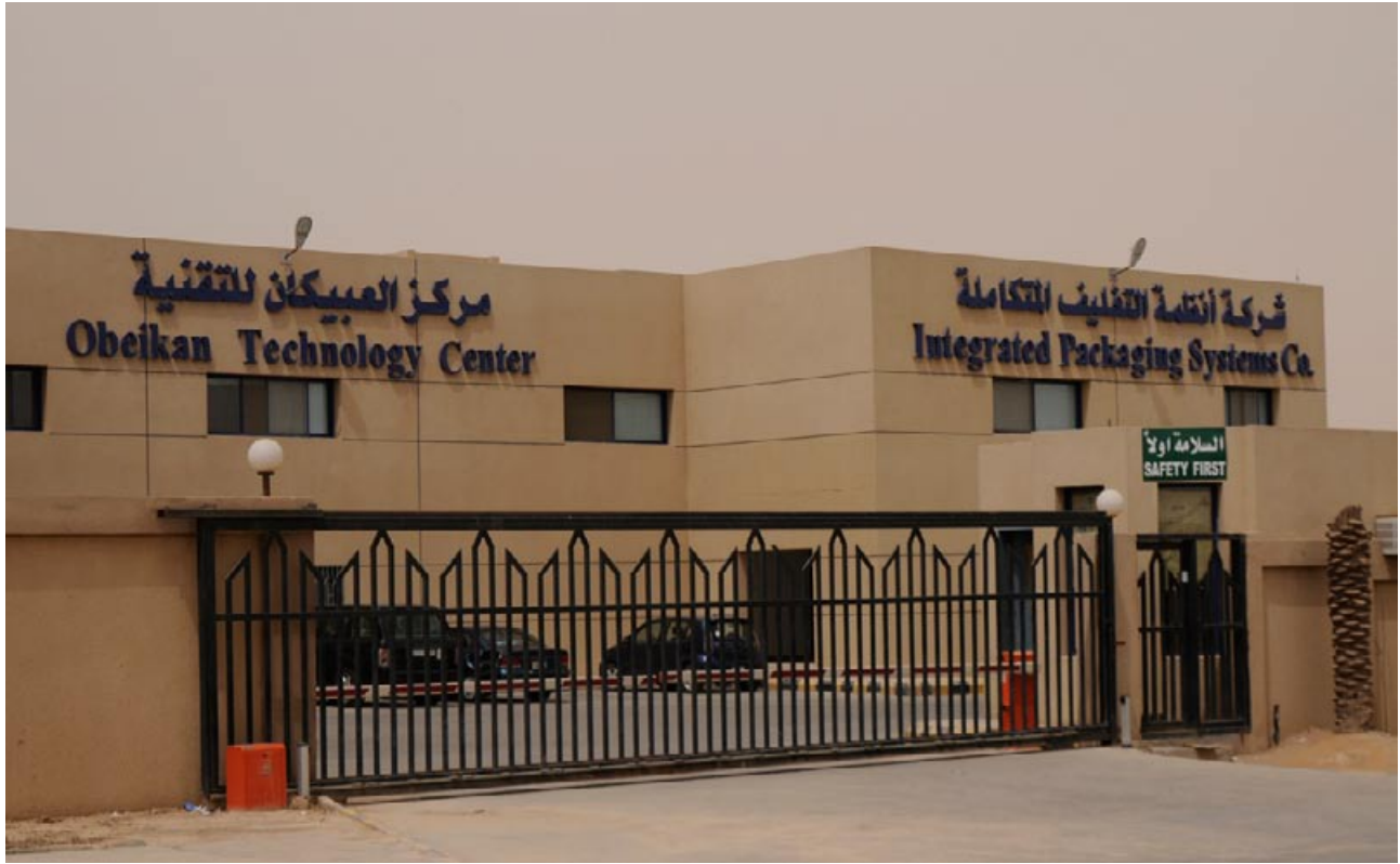
Obeikan Technological Center, headquarters front view, in Saudi Arabia.
