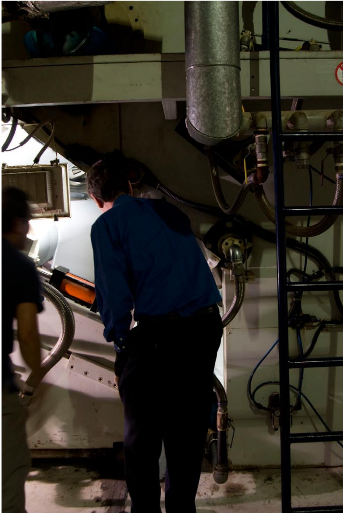
Gradually curiosity and interest in learning overcomes my hesitation to get inside the machine (realize the machine is in full production, with all heating units at full heat).
