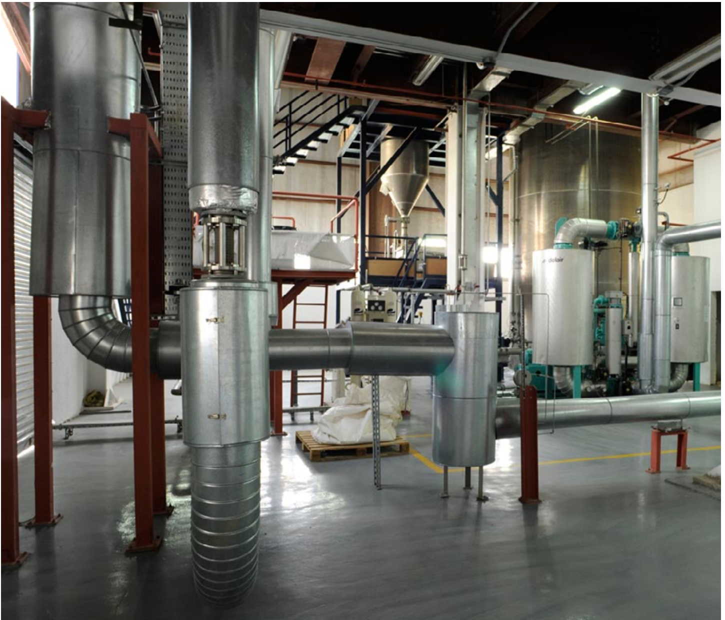
At the next level up (possibly the 7-meter level) I see the SSP air drying equipment. Notice the factory is clean and the equipment is top of the line (not cheap junk, and not jerry-rigged).
