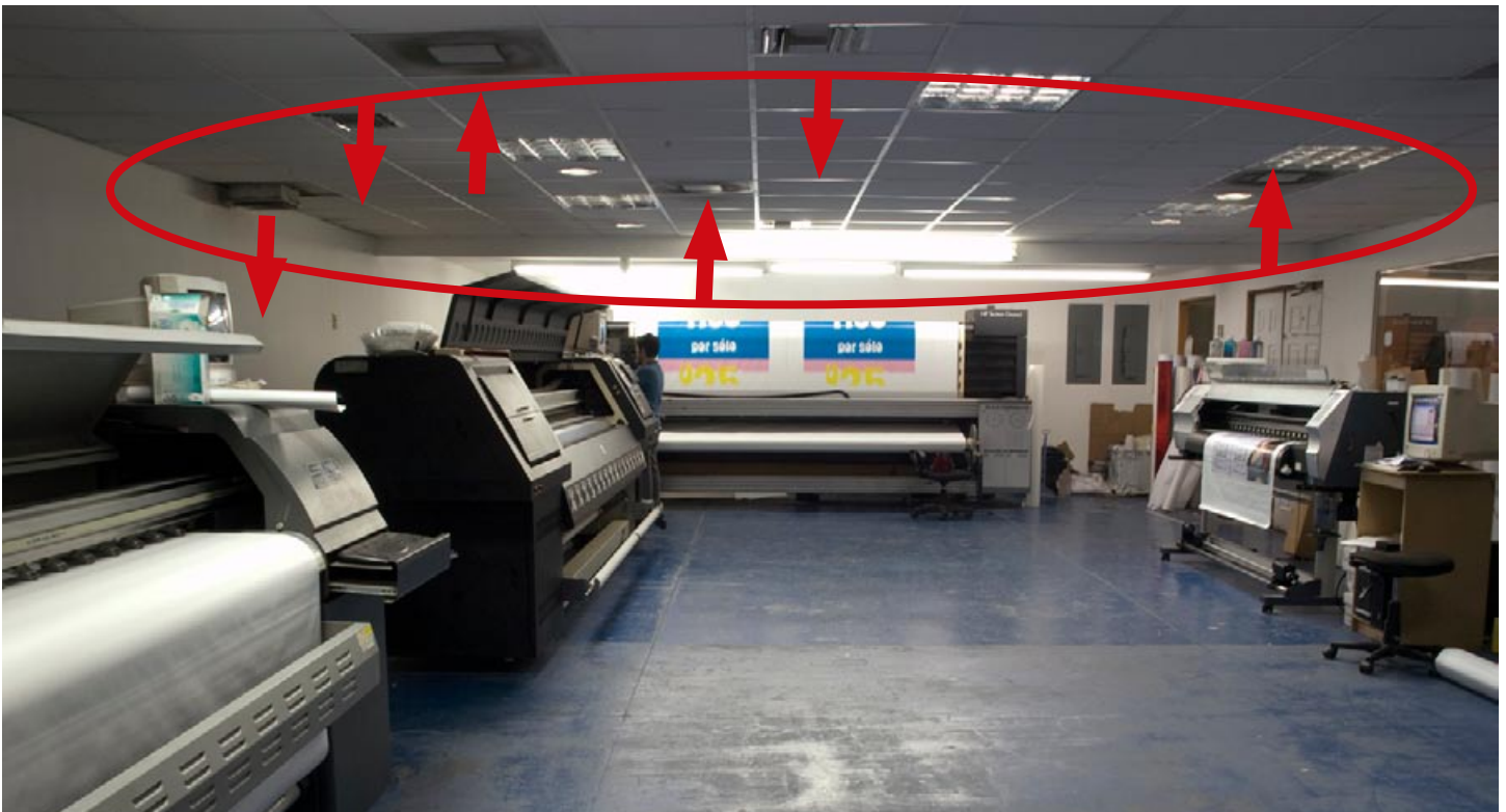
Print room inside view. In a solvent printer environment, it's necessary to have an air injection and extraction system, in order to have a controlled environment, free from the strong odor produced by the ink solvent. As the operators of these printers comments, since they made the change of ink, the solvent odor that AT Inks emit is not as strong as that previously used.
